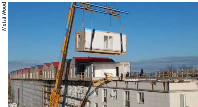
Figure 2.87. Light wooden extension floor to an existing multi-storey building from volumetric elements. Poissy, France.
