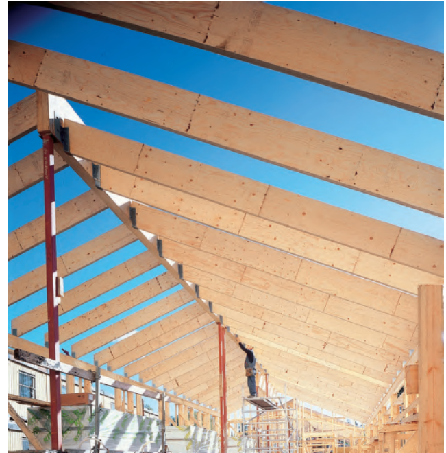
Figure 2.28. LVL-P rafters in a ridge roof structure.
