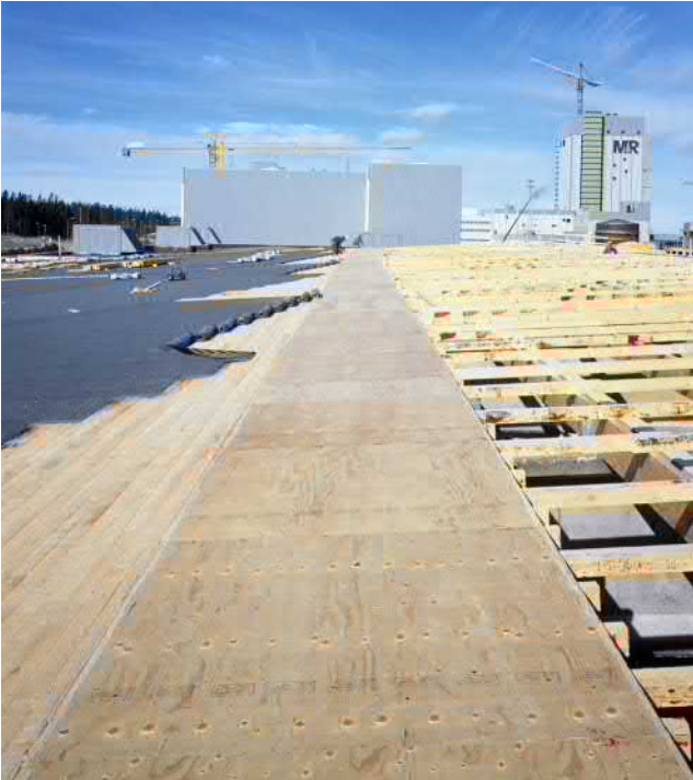
Figure 1.4 LVL-C roof panels.
