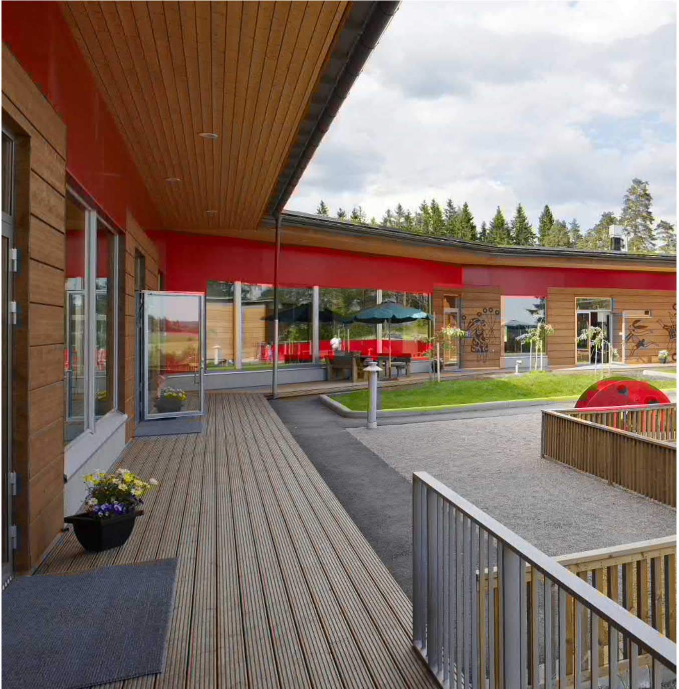
Figure 8.1 Roof overhang protects the building against weather exposure and solar radiation, Kindergarten Vekara, Pukkila, Finland.
