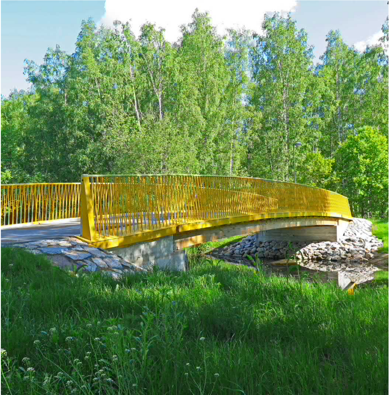
Figure 7.1. Wooden pedestrian bridge, Matinpuron, Espoo, Finland.
