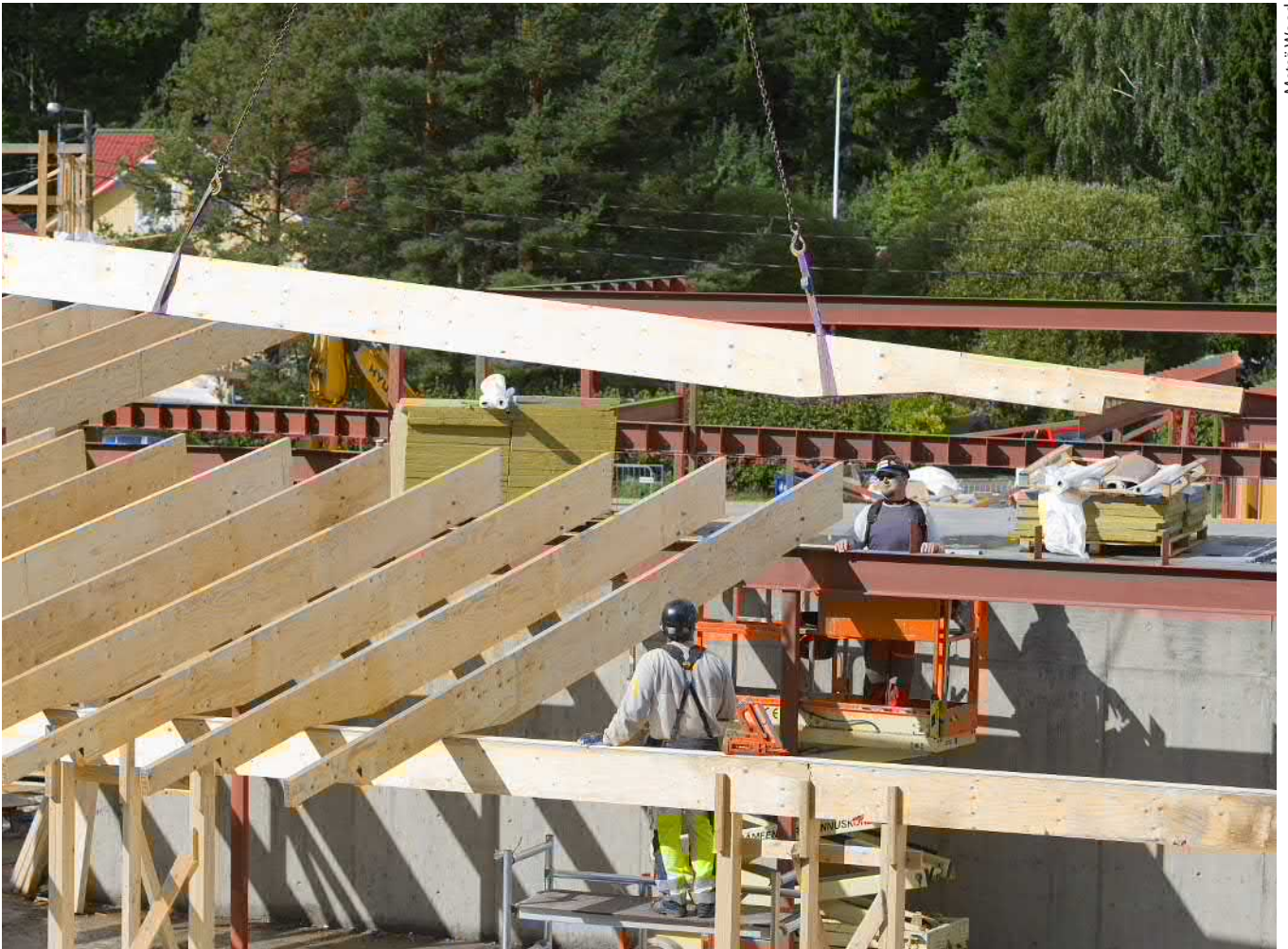
Figure 1.49. LVL-P roof beam cut to special shape.
