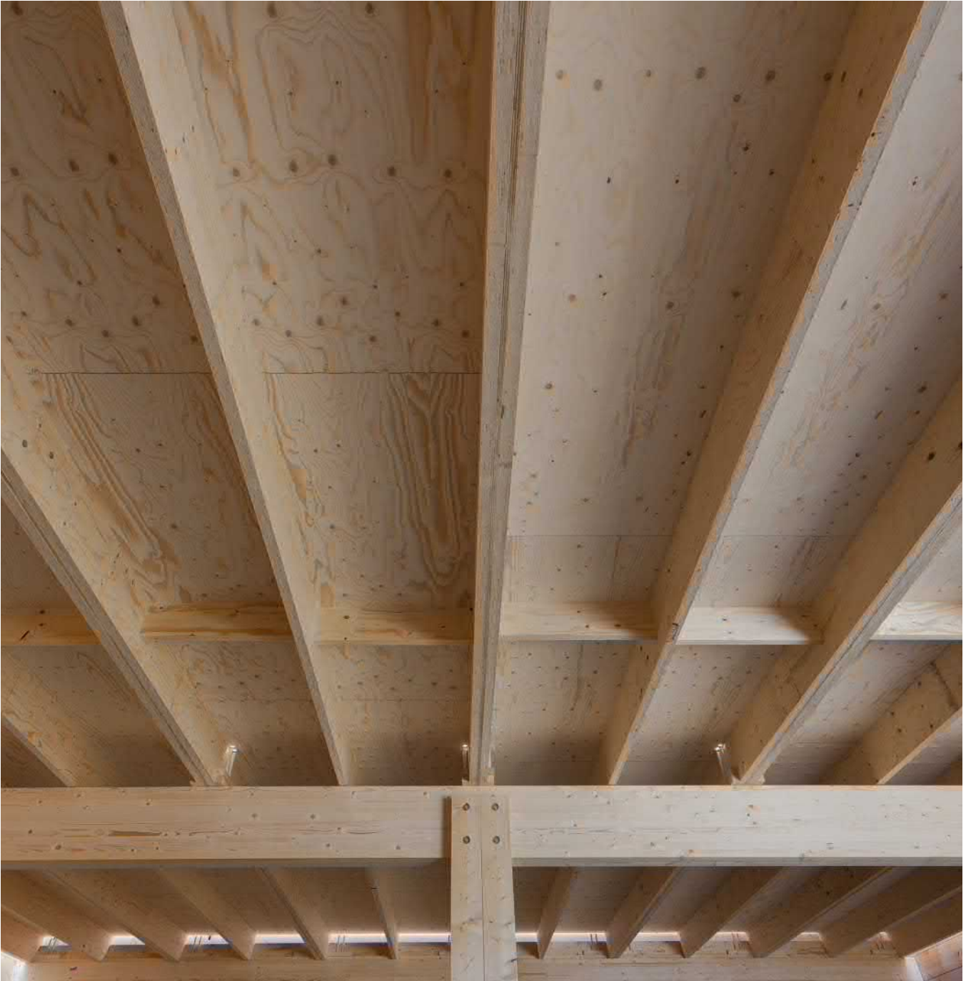
Figure 1.1 LVL roof structure, K-Rajamarket, Utsjoki, Finland.
