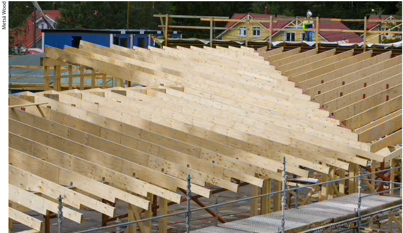
Figure 2.27. LVL-P rafters in a mono-pitch roof structure.
