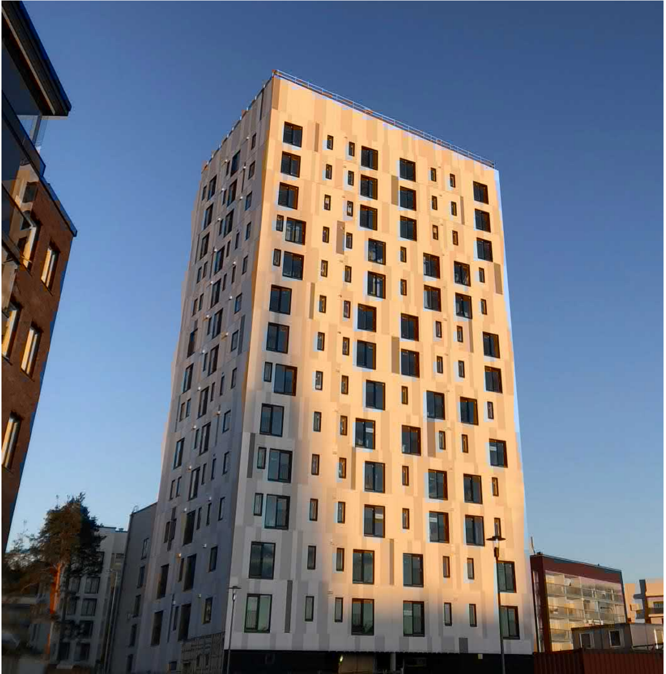
Figure 9.1. Wooden multi-storey building Lighthouse, Joensuu, Finland
