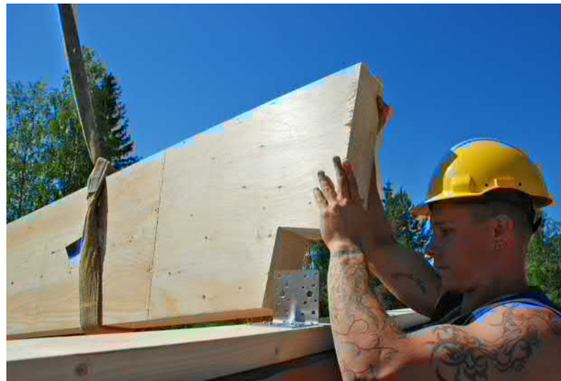
Figure 4.19. Installation of notched rafter beam.
