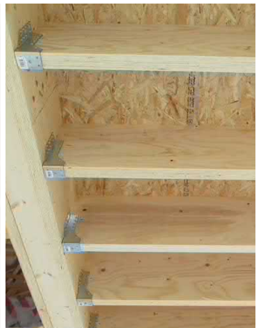
Figure 2.3. Joist hanger connections of floor joists.
