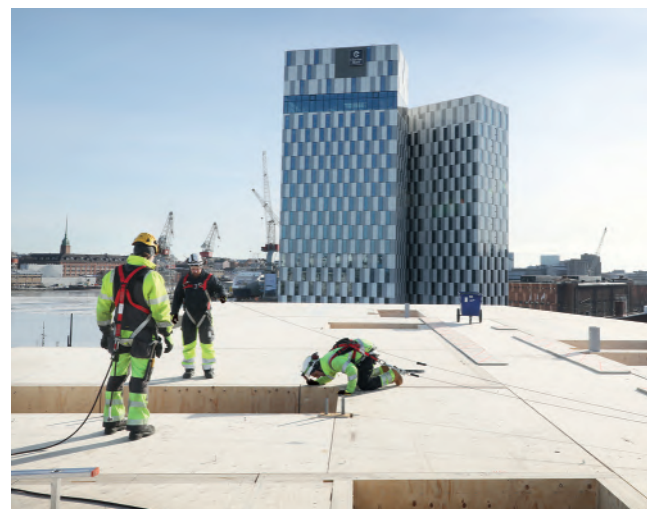
Figure 2.15. Installation of LVL floor elements.
