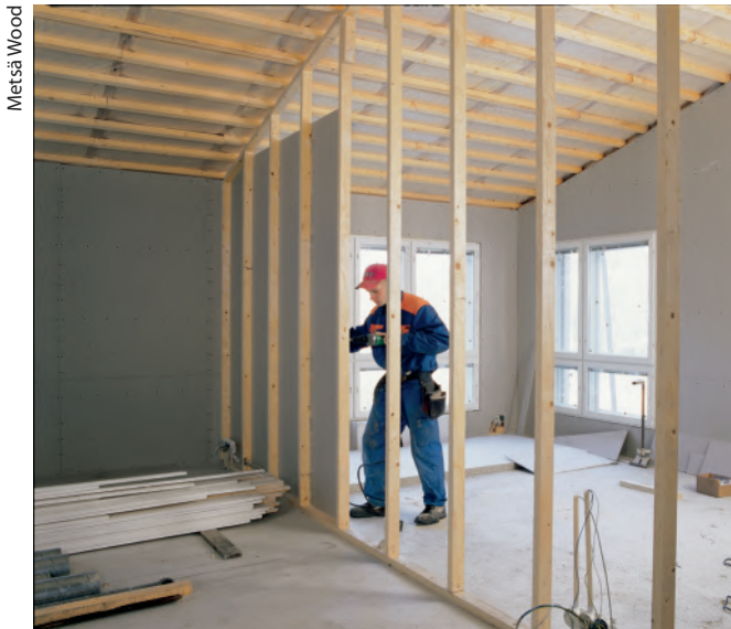
Figure 2.56. Installation of plasterboards to LVL-P wall studs.
