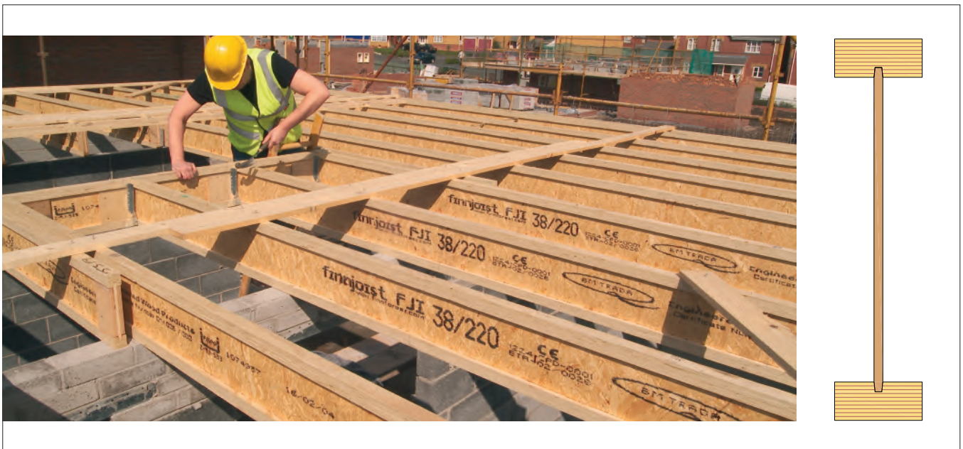
Figure 2.94. Wooden I-joist with LVL flanges.
