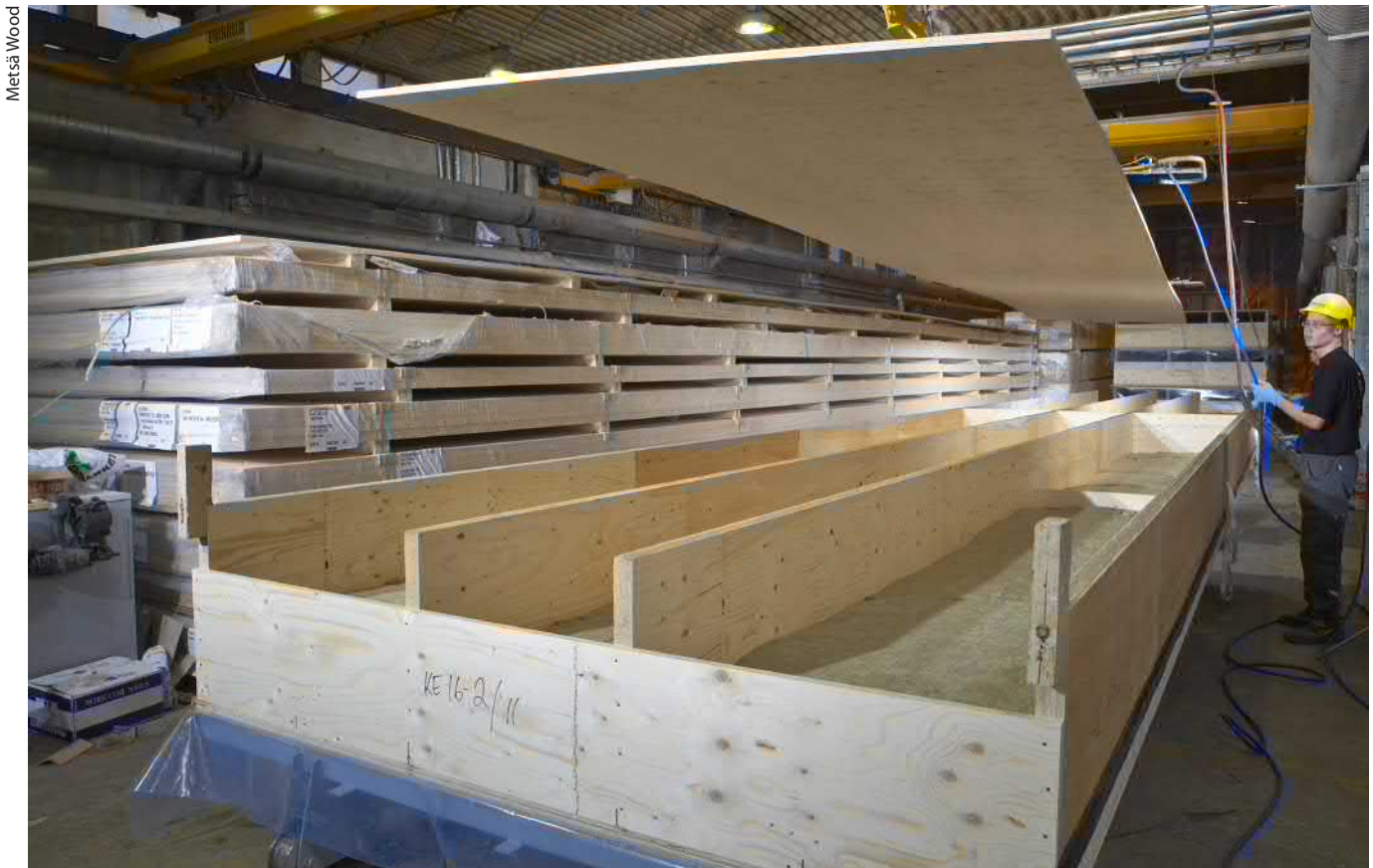
Figure 1.57: Manufacture of structurally glued LVL roof elements.
