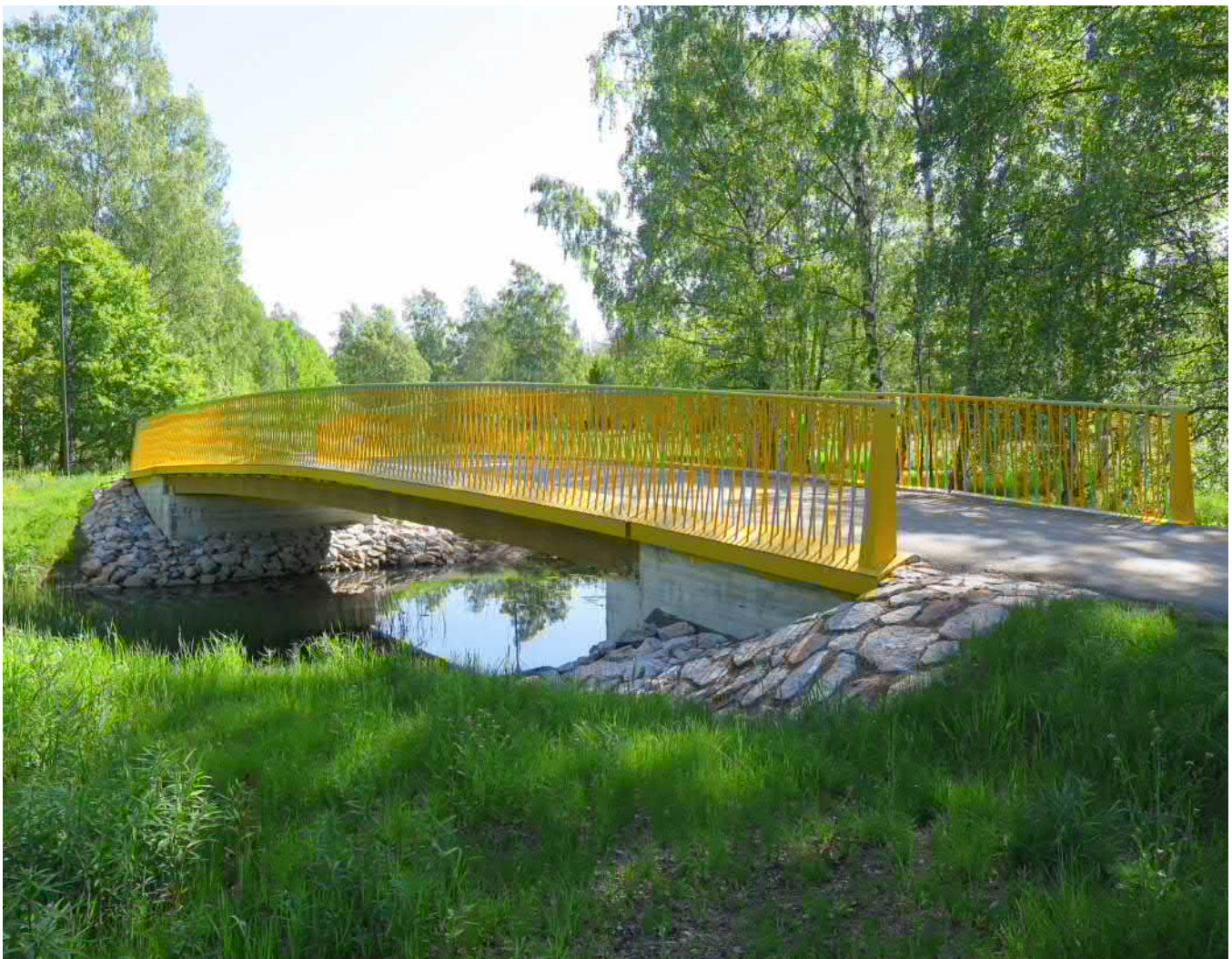
Figure 2.92. 75mm LVL-C deck on a pedestrian bridge. Matinpuro Espoo, Finland.
