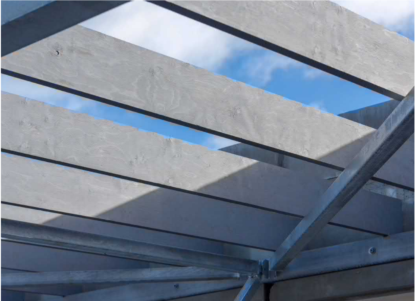
Figure 1.66. Coated surfaces of LVL beams.
