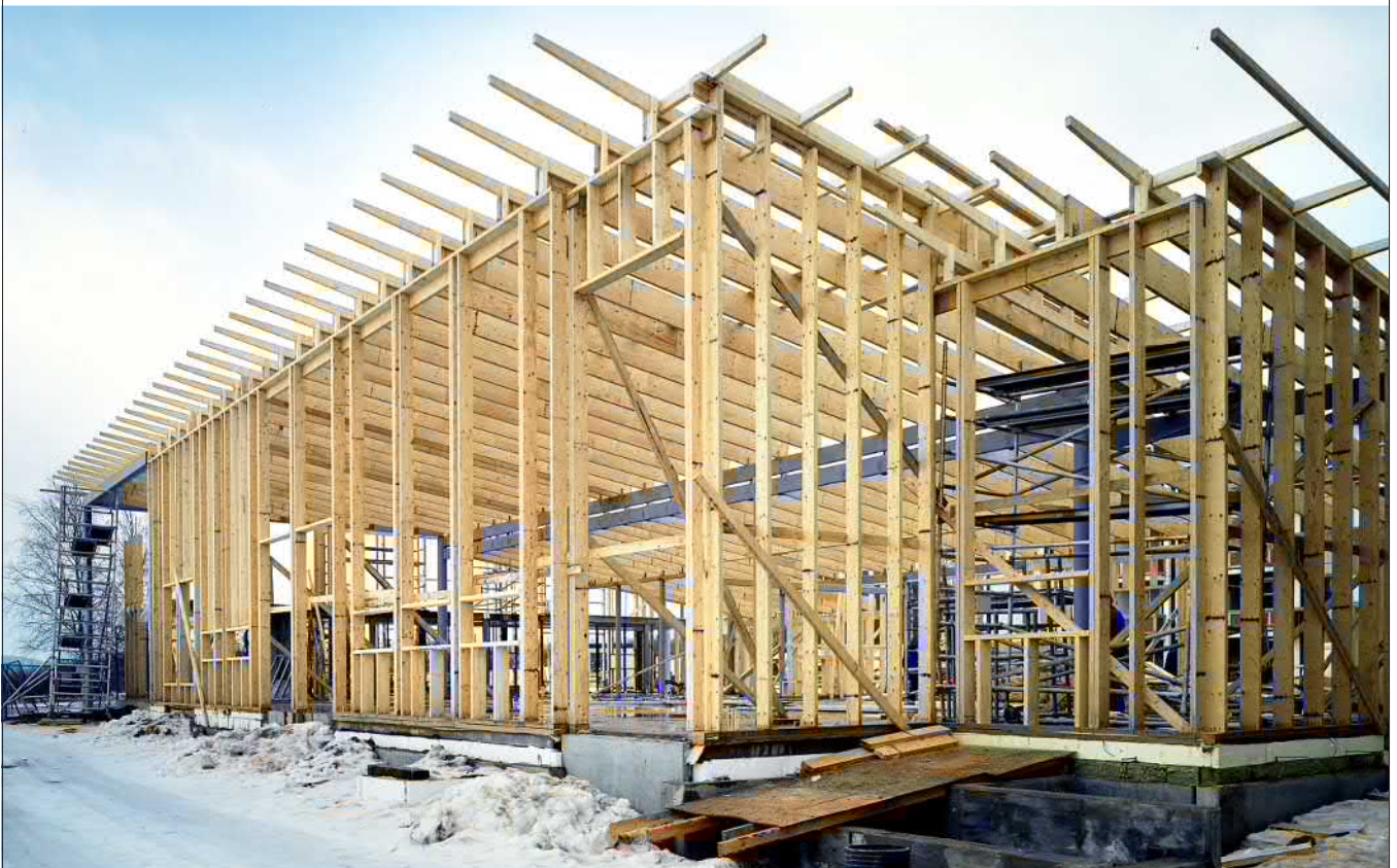
Figure 2.58. LVL-P studs for tall load-bearing exterior walls.
