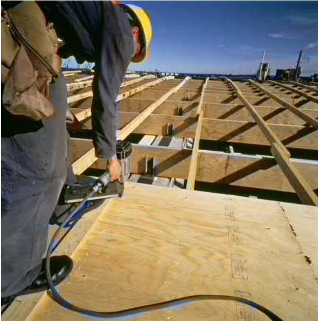
Figure 2.45. Installation of LVL-C roof panels.
