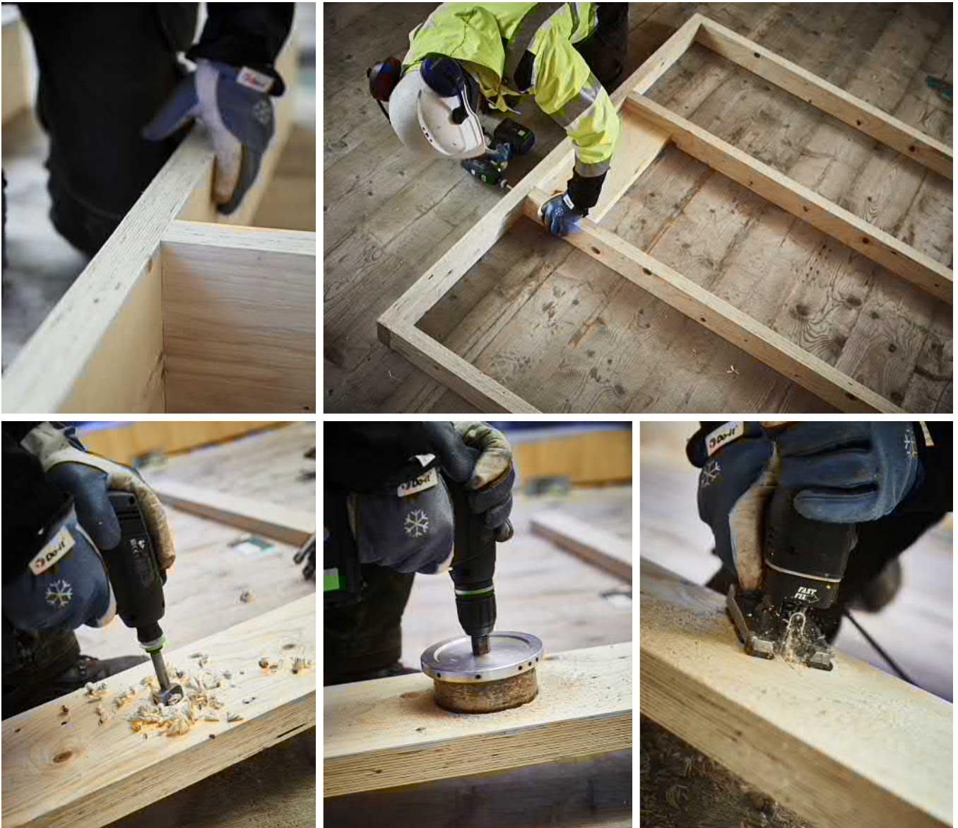
Figure 3.6. LVL structures can be processed with conventional wood working and power tools.
