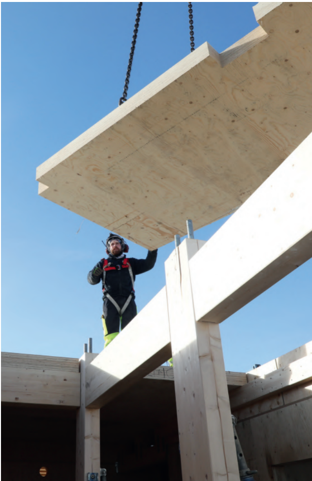
Figure 2.13. Installation of a multiple-glued GLVL-C floor element.
