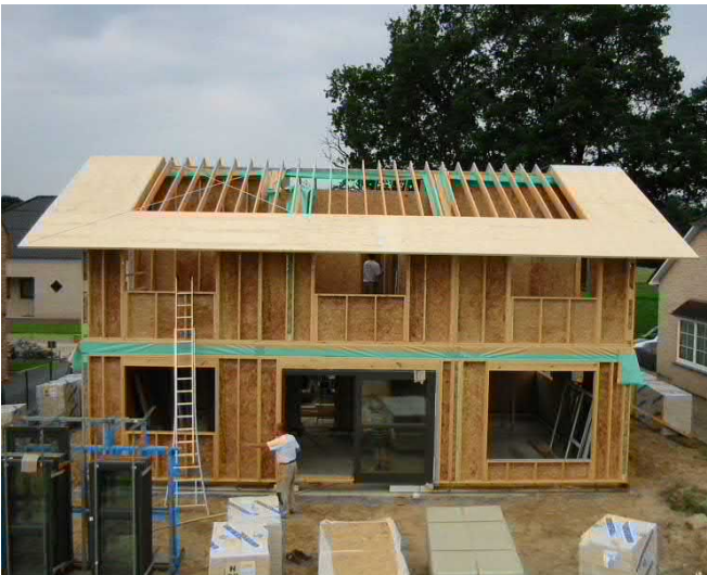
Figure 2.47. Eaves and roof overhangs from LVL-C panels.
